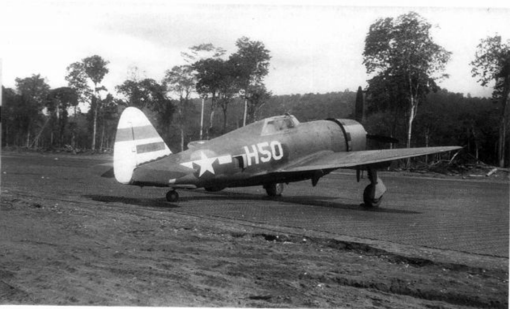
* H50 was a P-47D assigned to the 310th FS, 58th FG at Dobodura, New Guinea. The cowl, tail band, and possibly the canopy frame are painted yellow. The Jug sits on a pierced steel planking (PSP) ramp. PSP kept the ramp and taxiways from turning into a quagmire during the rainy season. (E.M. Sommerich via P.M. Bowers)
