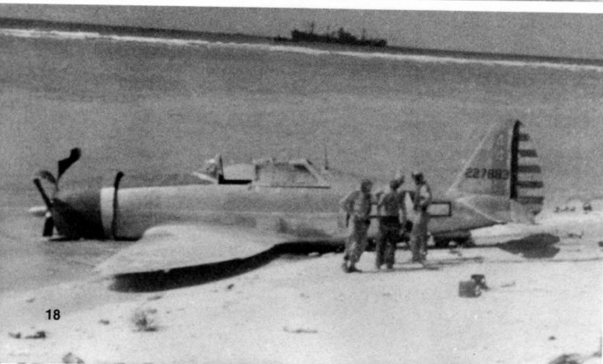
This P-47D-23-RA (42-27883) hit a C-47 transport while taking off at Tarakan. Both the pilot and the slightly bent Jug wound up on the beach. The aircraft wears the red cowl and vertical fin band of the 341st FS. The aircraft number (44) is painted on the fin band. The lack of black ID bands indicate the incident likely occurred prior to November of 1944.
